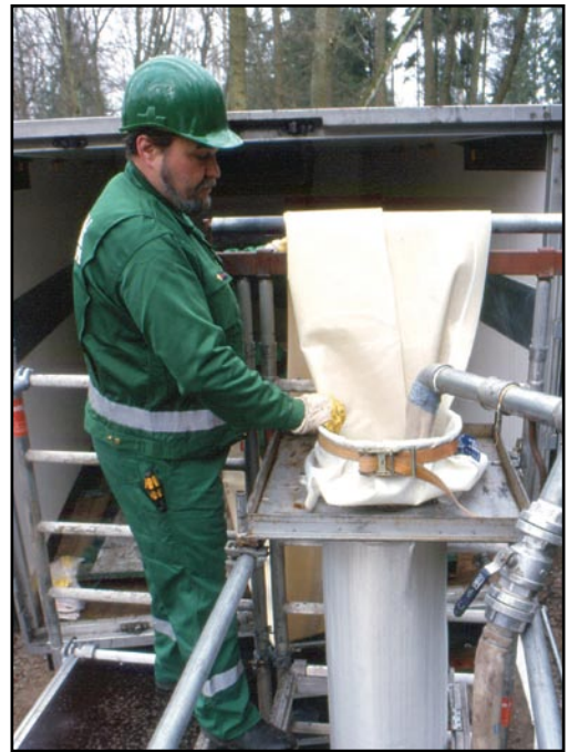
Trenchless sewer repairs using the KM INLINER ® system used successfully throughout the world since 1980 by KMG International of Germany
